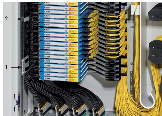
Recommended positions of conduit bracket (1) and retainer for cables and conduits (2)
