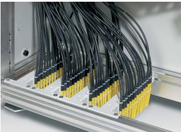
Cable tie plates with simplex loose tubes
