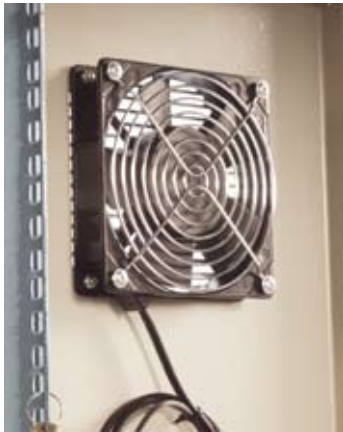
side panel installation
